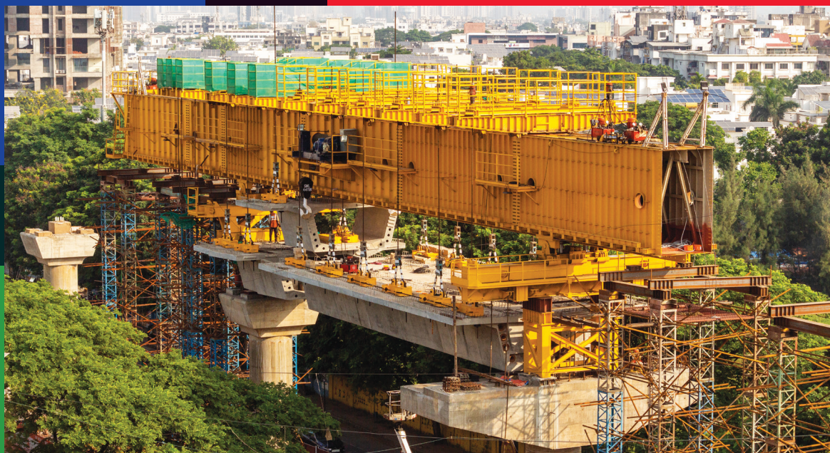
Viaduct works and launching of beams - Surat metro project, India © Bhoomi Gondalia / AFD
